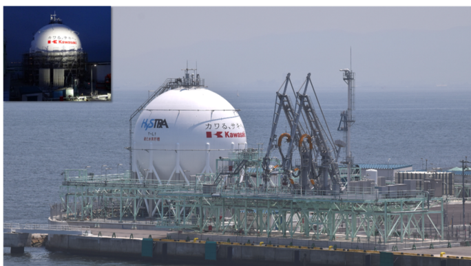
Wasserstoff-Terminal Japan, Kawasaki Gas Turbine Europe
