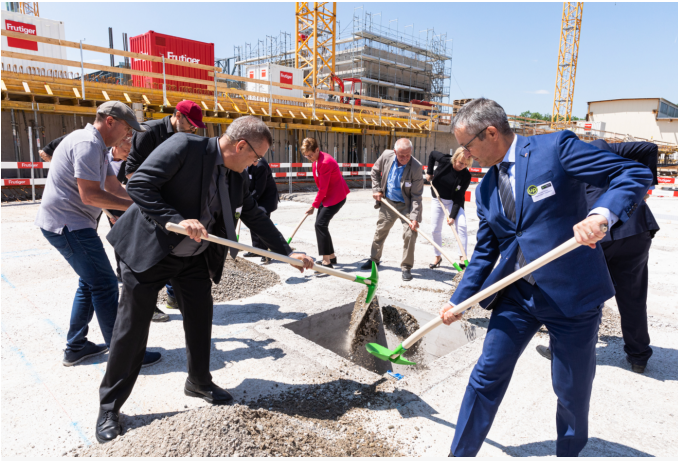
The official laying of the uptownBasel foundation stone took place on 7 June, 2019.
