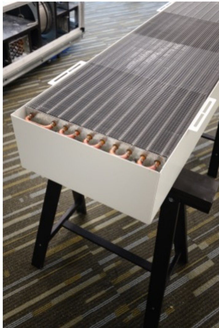
Passive chilled beams
